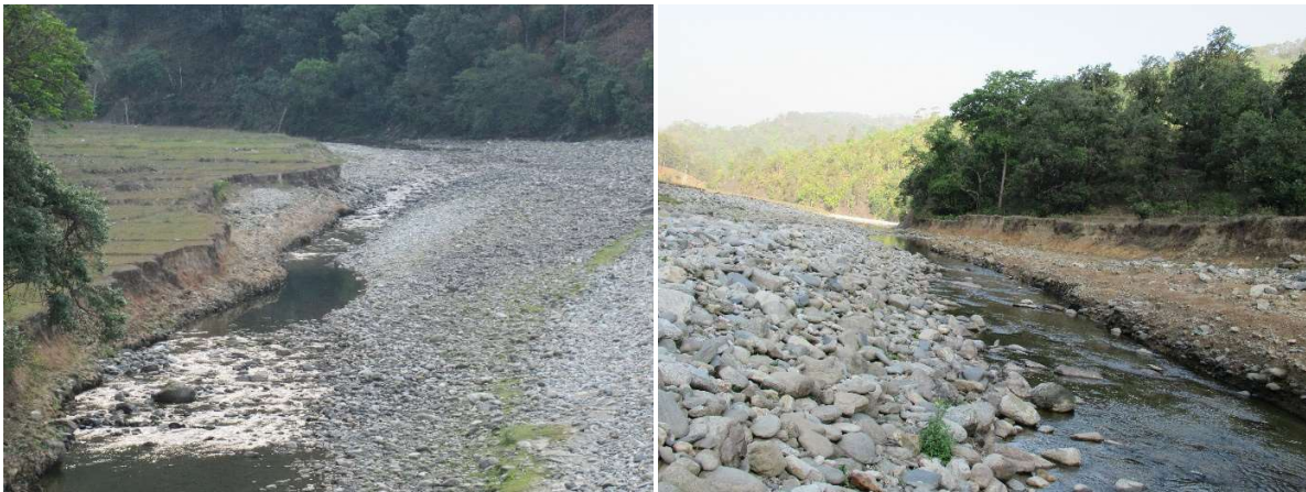
Photo 1: Toe cutting by river bank cutting at Deuli
